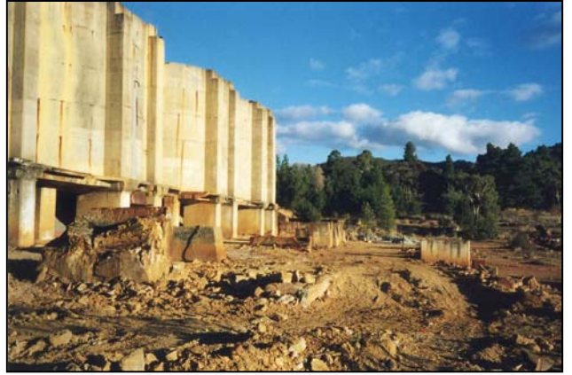
Storage Bins and Ball Mill. Photo – Barry McGowan 2006
