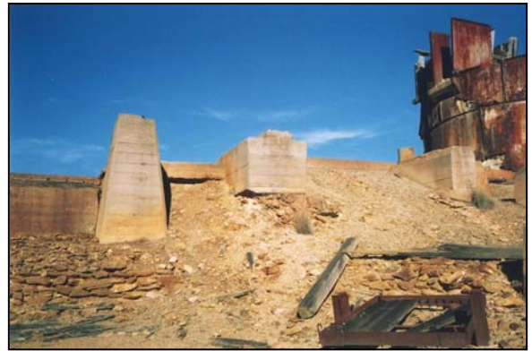
Surge Bin & Associated Structures. Photo – Barry McGowan 2006
