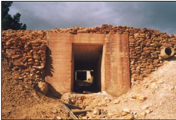
Waste Drain – Northern Site. Photo – Barry McGowan 2006
