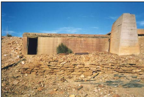
Store Room Below Surge Bin. Photo – Barry McGowan 2006
