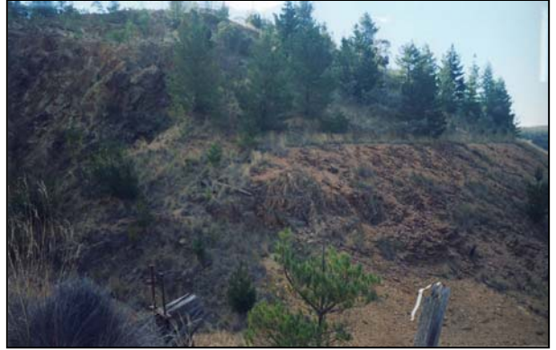
1890s Railway embankment. Photo – Barry McGowan 2006
