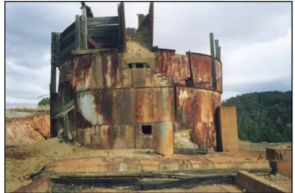
Surge Bin. Photo – Barry McGowan 2006
