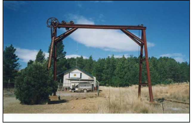
Gantry & Railway Store. Photo – Barry McGowan 2006
