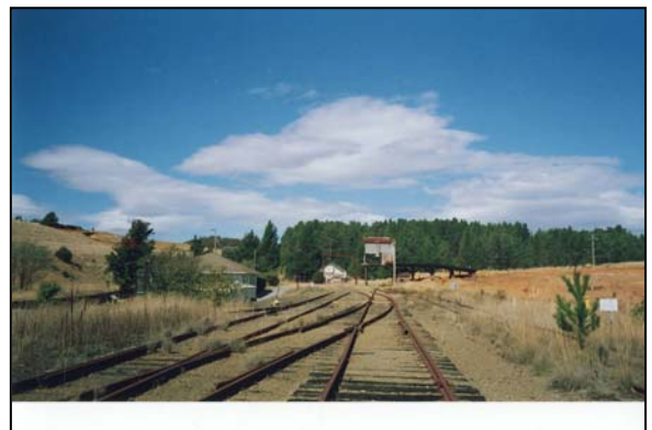
Railway Complex. Photo – Barry McGowan 2006
